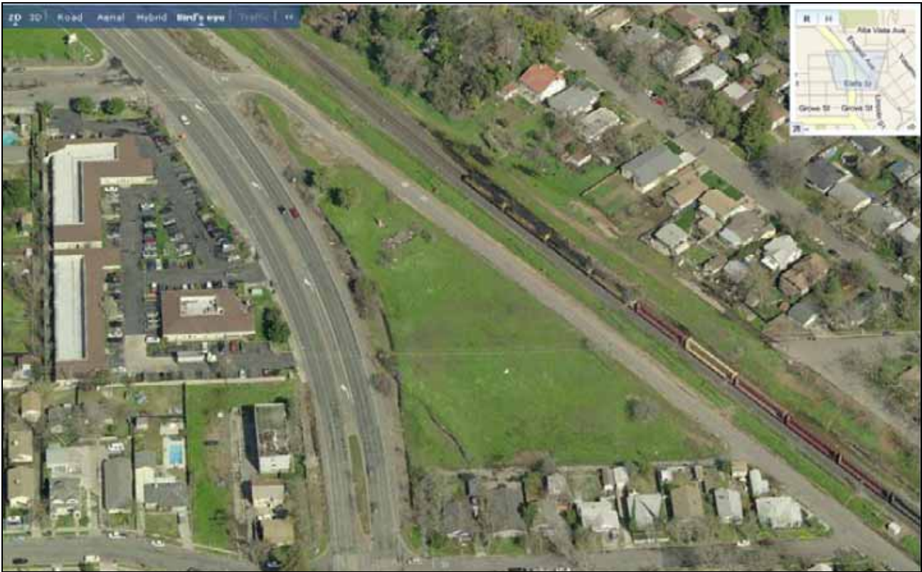
Figure 4.9. View looking north of Washington/Lincoln Catalyst Site (from Virtual Earth, Microsoft Corp.)
